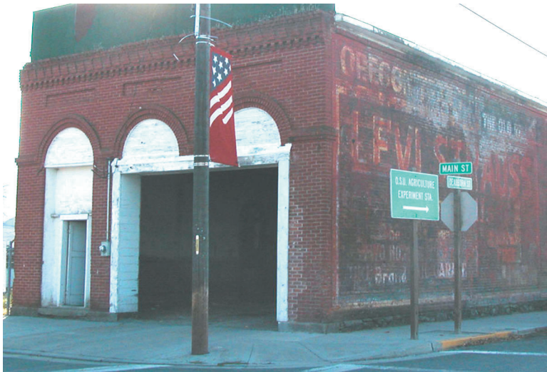
This is a building from the late 1800s that was built for a brewery. It has about a dozen signs painted on the side. Dave Kent, who lived here years ago, was a sign painter and painted all these signs. There was a garage there in the 1920s, and it's now used as a bus garage. The foundation is rocks piled up, similar to many of the old buildings; they didn't have cement, I guess.
